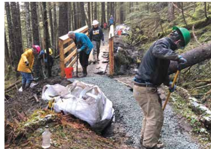
New Treadwell Ditch Trail bridge
